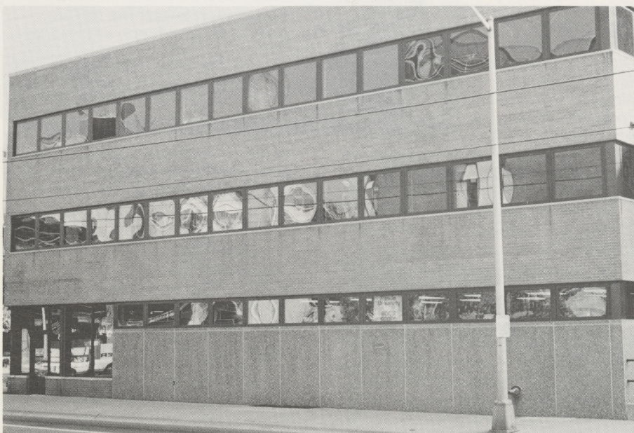
New windows add to exterior aesthetics. ▼
